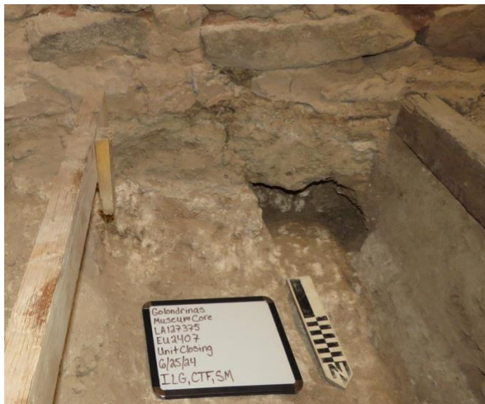
Figure 21. Closeup of globules of lime. The lime globs run under the apron and up the exterior wall.
