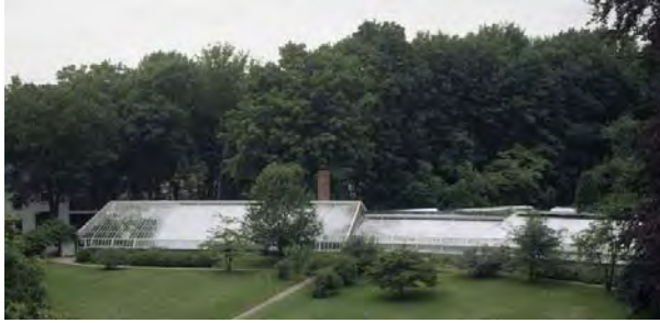
Figure 3.7. Overview of the Lyman greenhouses at the Vale, Waltham, Massachusetts.
