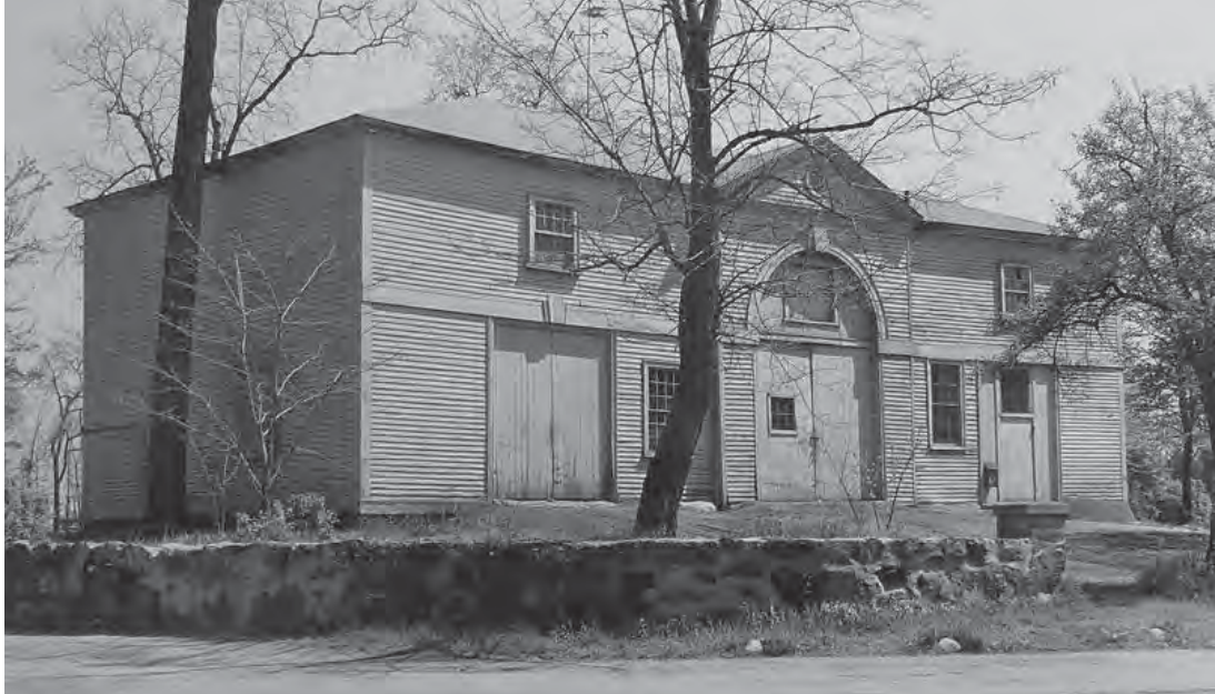
Figure 2.1. Carriage house as it appeared ca. 1937.
